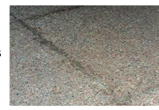
Divider strips can bleed color as they are polished dry. Divider strips are made from aluminum (epoxy terrazzo only), zinc, brass or plastic.
